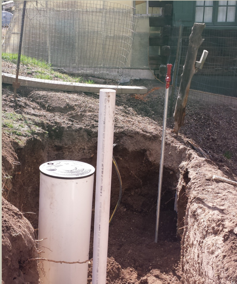
FIELD INSTALLATION Frost Free Hydrant Installation
