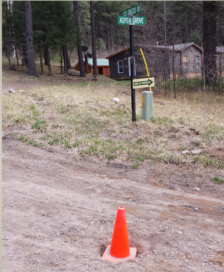
FIELD INSTALLATION Phantom Cone --- Leaking Isolation Valve
