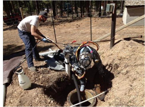
Figure 9. Entering Tank 3 while being decontaminated with chlorine solution. Tanks 3-5 and 1 had 22 inch diameter hatches.
