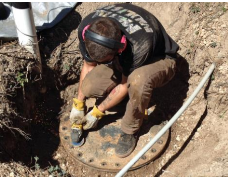
Figure 7. Cutting Off Tank 3 Bolts in System 1.
