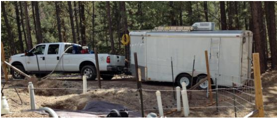
Figure 6. MDS truck and trailer lab at System 1 to inspect Tanks 3, 4, and 5. We believe these tanks hadn't been inspected for many year judging by the rust on the bolts holding the tank covers closed.
