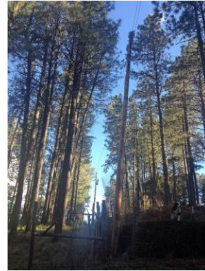
Figure 3. Trees over power line at 84 Hovenweep Loop.
